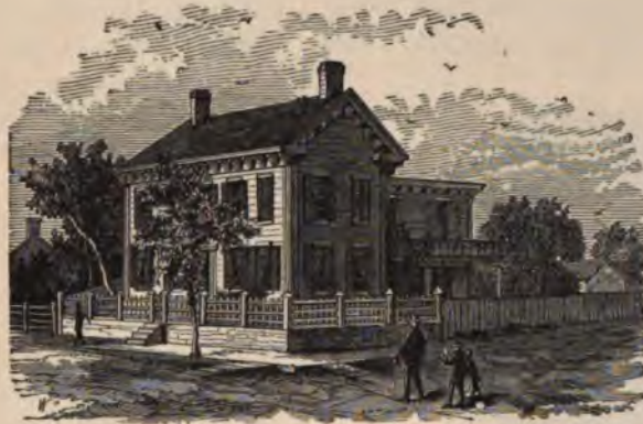
LINCOLN'S RESIDENCE AT SPRINGFIELD, ILL.
